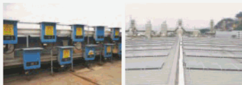
Location: Rooftop of Canadian Solar's factory Capacity: 1.2 MW Inverter: 53 x GW17K-DT, 20 x GW15K-DT
